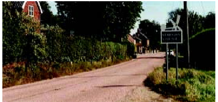
Before and After - Natural traffic calming in Norfolk At Starston, signs and centre lines were removed and a bespoke gateway sign introduced.
